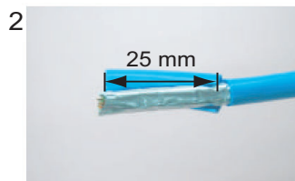
2 Remove the outer sheath by approx 25 mm. Be careful not to damage inner shield and cores.
